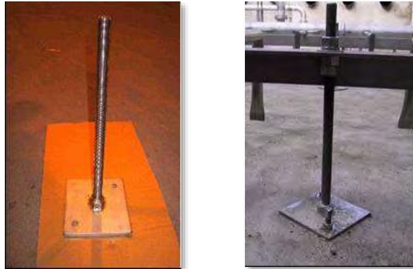
Outside Diffuser Support
