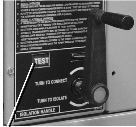
Figure 3-17. Isolation Handle turned to TEST .
