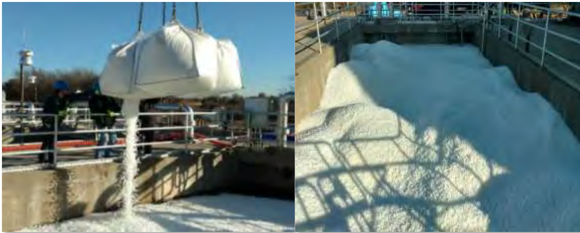
Media Installation into Reactor & Pouring Media into Reactor
